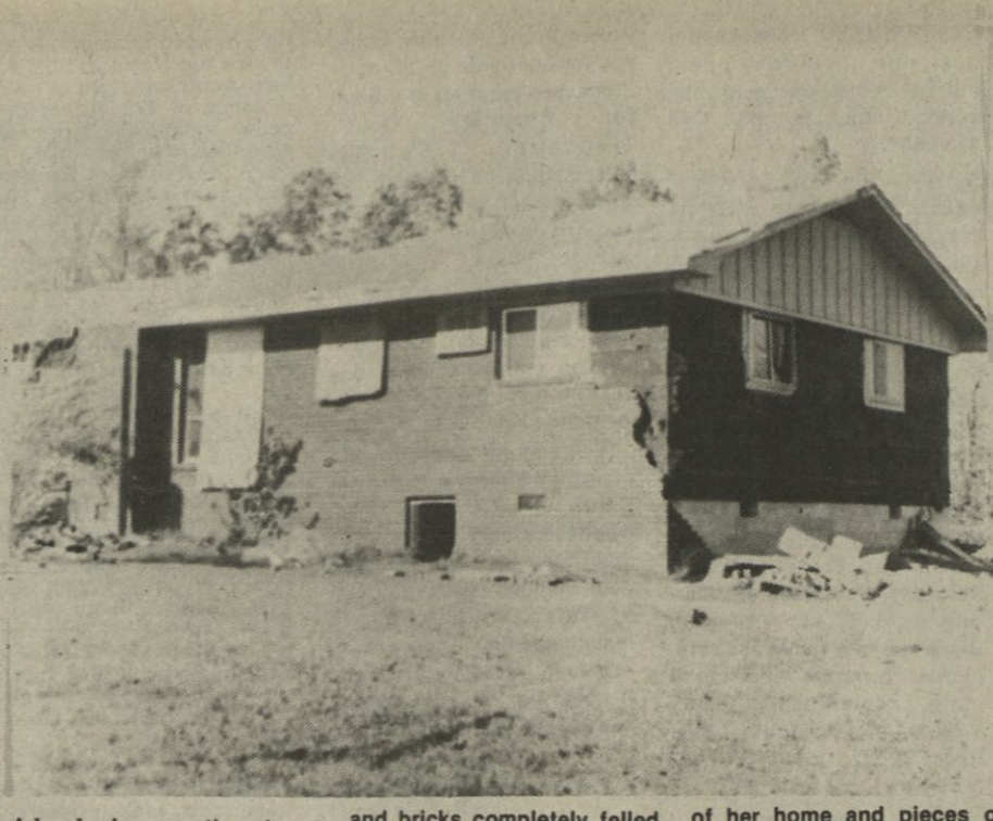
A back view, south and east sides, of Jackie and Jane Dean's house following last week's storm shows where the chimney top was blown away, windows shattered out, and bricks completely felled from the house portion. The Dean's were not at home during the impact. Mrs. Dean reported glass had to be "scooped" from the interior of her home and pieces of glass embedded in the walls and inside furnishings. A favorite chair for relaxing belonging to Mr. Dean and the one he normally sits in was split in half, she said.
