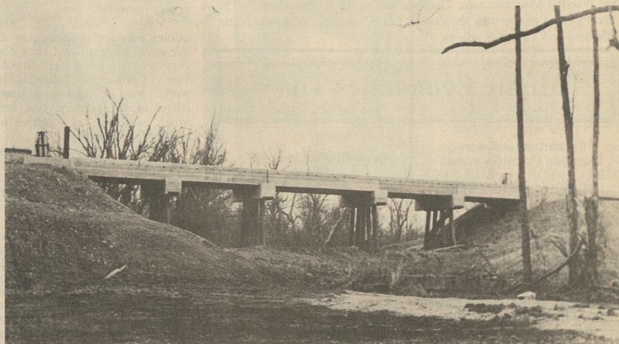
Railroad Trestle Now In Use — This newly completed trestle over Indian Creek in Iuka was built by Norfolk Southern Railway at a cost of about $500,000. A culvert system, used for many years, is believed to have aided in the flooding of Mineral Spring Park and the surrounding area.
