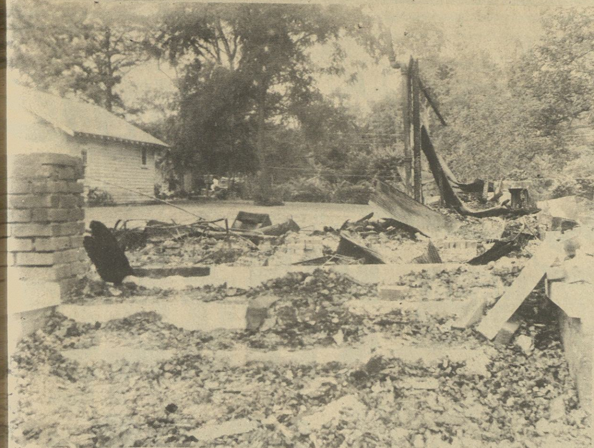
DESTROYED BY FIRE... two-story home of Mrs. Whitaker was recently destroyed by uncontrollable fire Friday night, July 6. The large house, located at West Second Street in Burnsville, Tishomingo, was approximately 100 years old and Mrs. Whitaker resided there for the past 20 years. According to Iuka Fire Department records, the fire started in the second story of the
