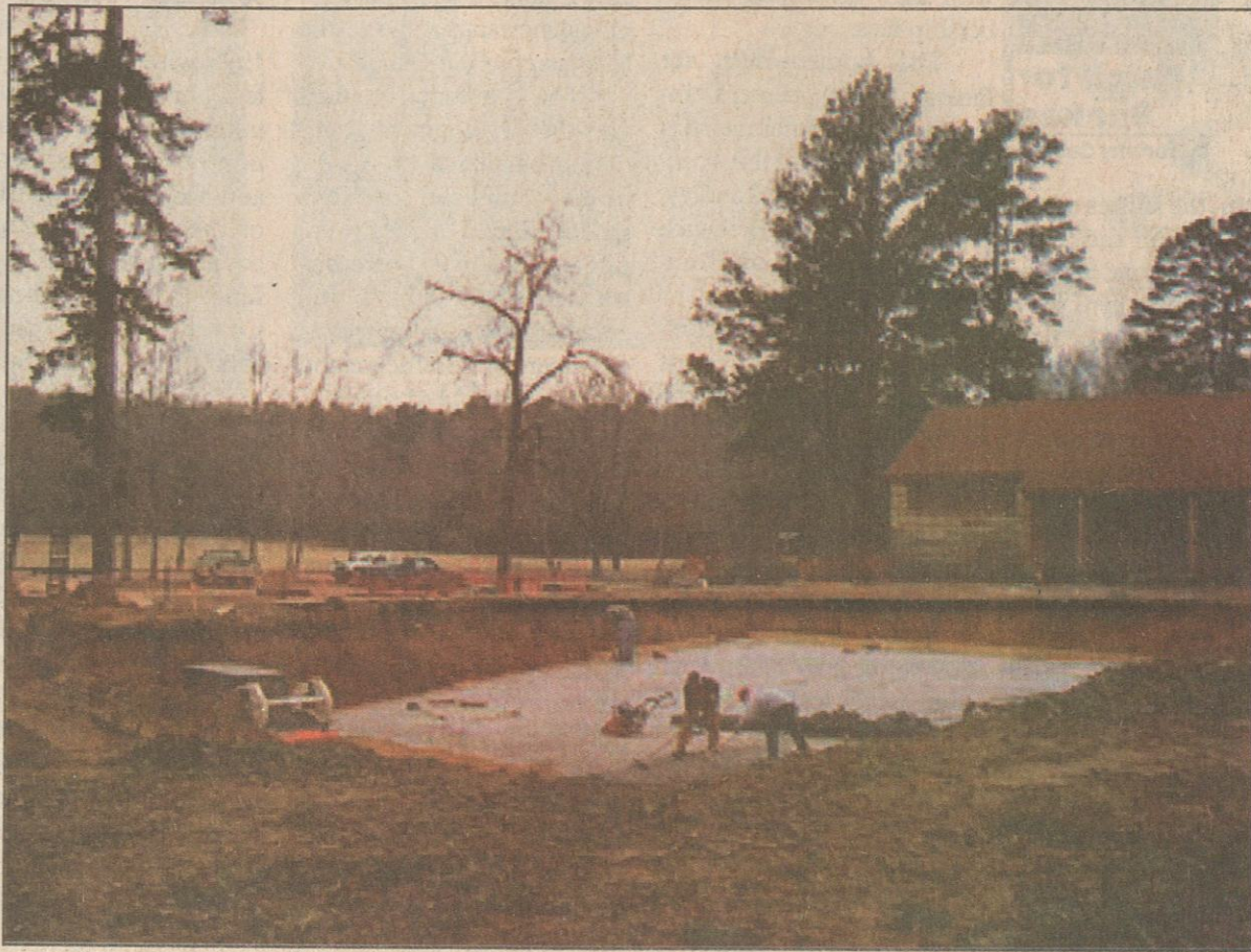
New Pool! Workers put down a base of limestone in the hole that will soon be Tishomingo State Park's new swimming pool. The building at right is the existing pool house.
