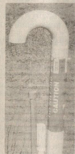
Pipeline Casing Vent
