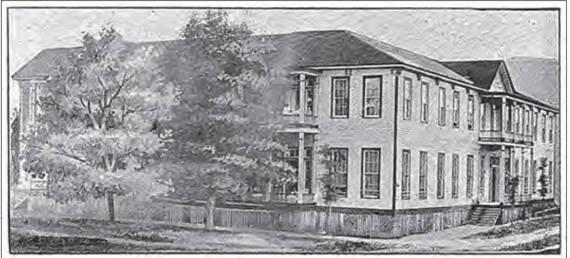
THE DORMITORY. The property of Iuka Normal Institute Co.
